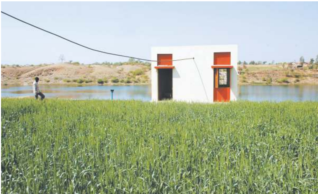
A pump house in Banswara, Rajasthan
