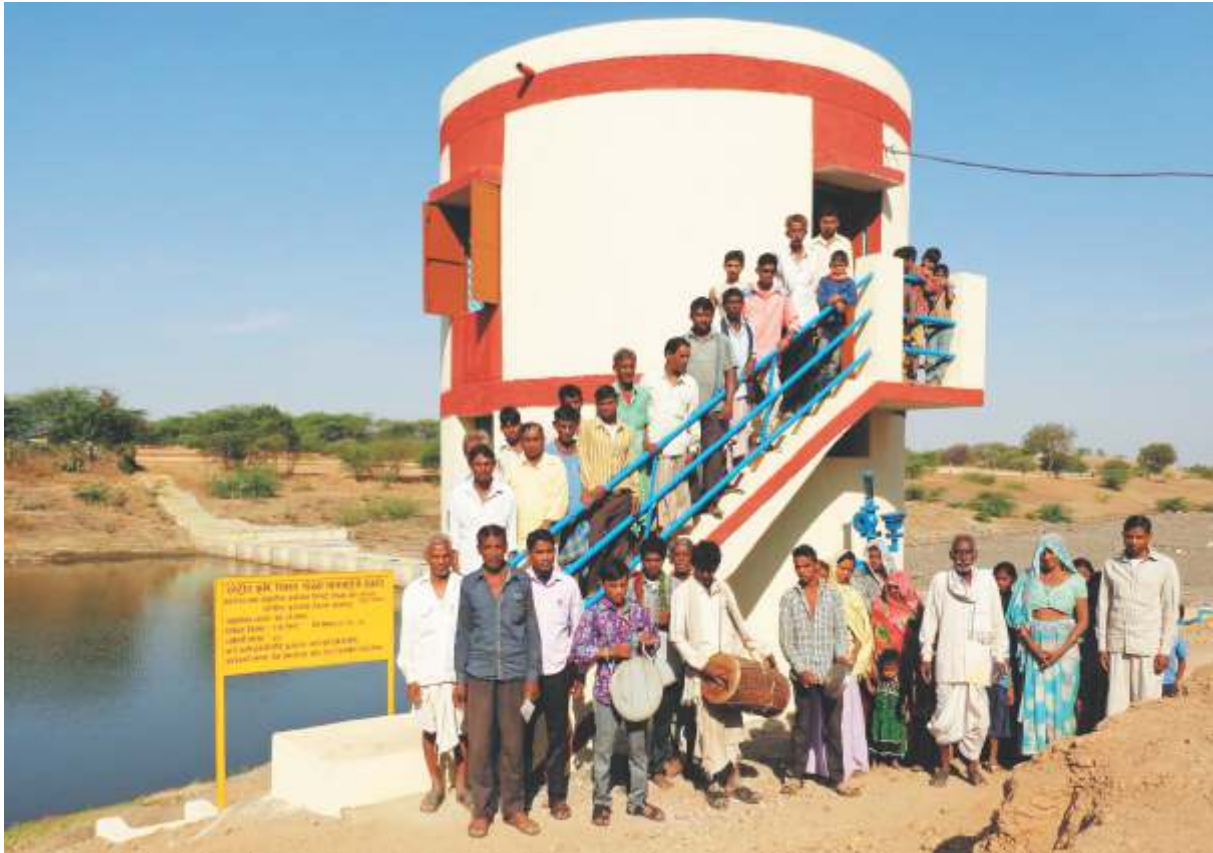
LI distribution Pump House, Borkhedi in Banswara, Rajasthan
